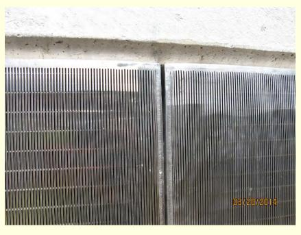
Fish screen panels constructed of V-wire profile bar with <0.0689-inch width openings
