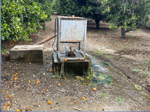
Artesian Well near Boardman and Ojai Avenue
